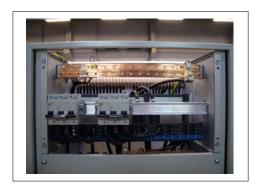
The standard AC output distribution unit is designed with a 35 mm DIN rail, Multi Clip termination board and N/PE copper terminal bars, and built as a part of the cabinet.
